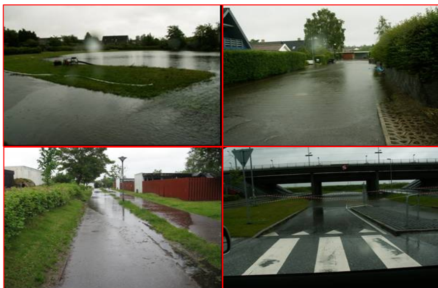
Figure 11: Aspects of the physical damages in Egedal on 13-06-2009.
