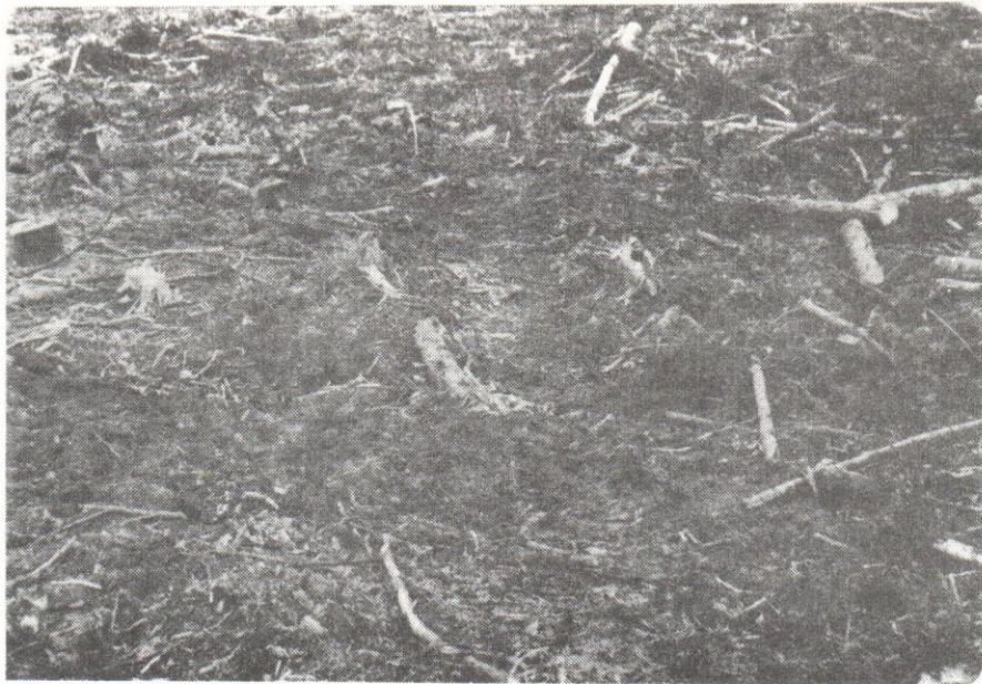
Figure 30 . Site Cleared by Crosswise Raking. (Compare Figs. 1, 16, 22)
