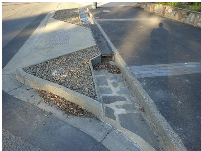
Different gutter crossing (plastic grate) and mulch (crushed slate) introduced at Aldinga Road
