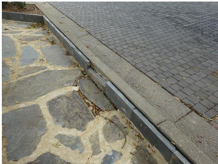
Concern that vertical slate tiles may delaminate over time, no protective capping
